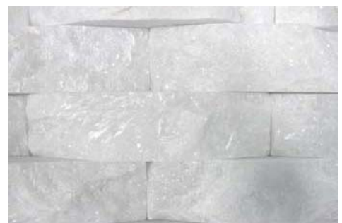
Asbestos-containing decorative stack-stone wall tiles
